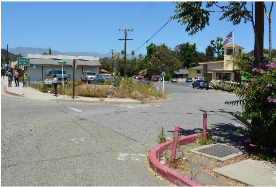
Figure 2: Highway 33 and Park Avenue; non-ADA compliant ramp, and inconsistent sidewalk network.
